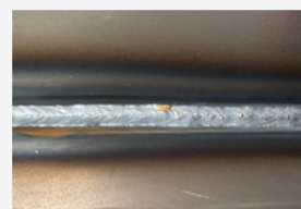
WELDING OF THIN SHEETS
